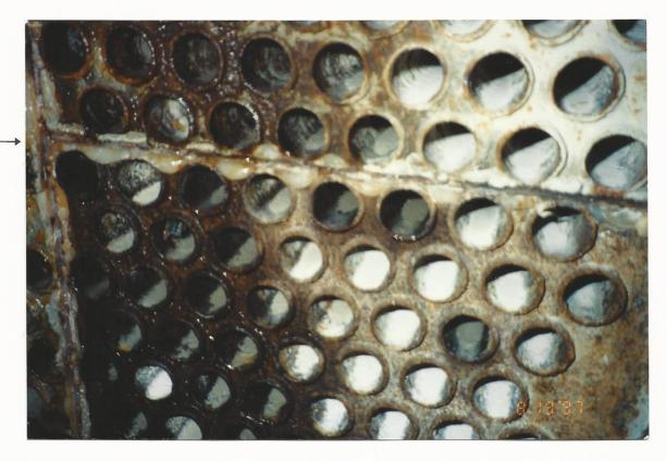
Magna-Tek Water Conditioner & Descaler installed August 1997 (after cleaning)
